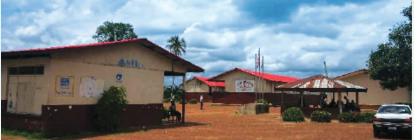
SDPL Central High School in Senjeh District, Bomi County
